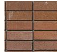
STACKED BOND BRICK CLADDING
